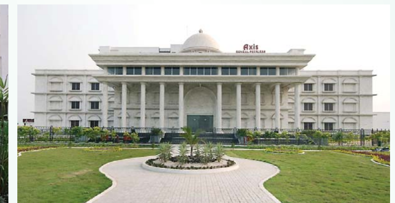
Commercial complex : Axis, Rajarhat, Newtown
