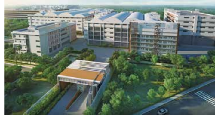
SRIJAN INDUSTRIAL LOGISTIC PARK On NH 6
